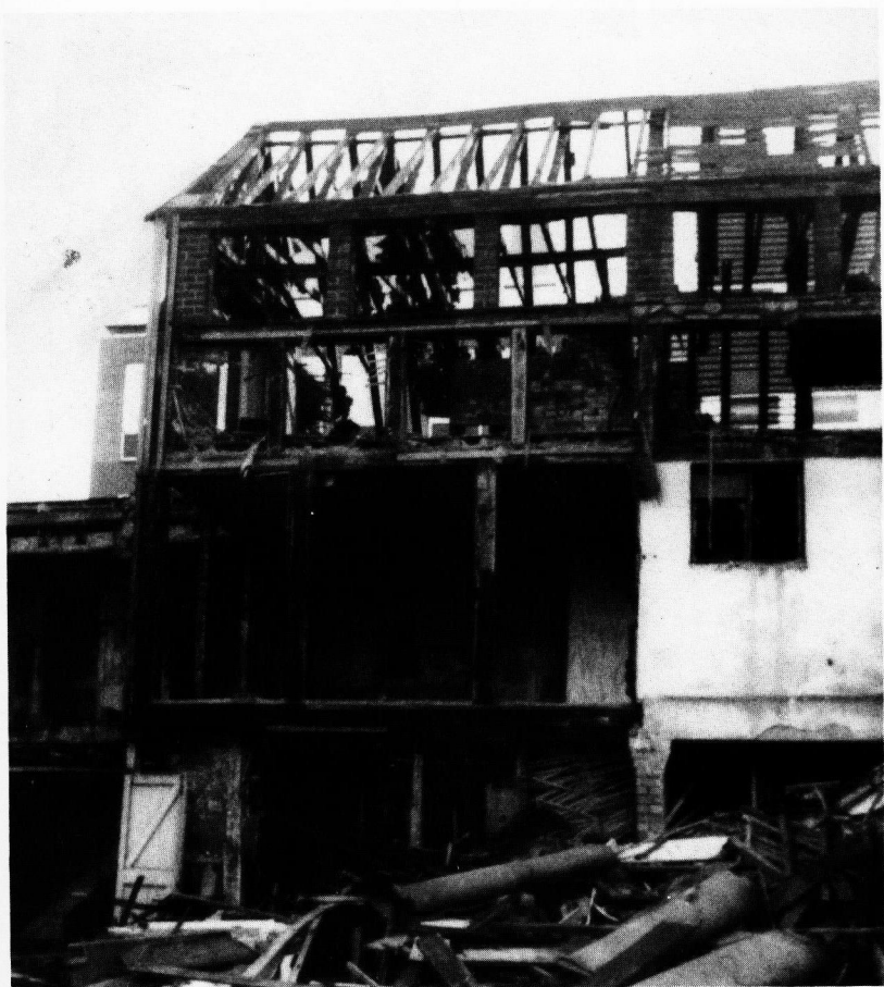
The jettied north wall of 17—19 London Street, with its timber framing surviving in good condition on all floors. (Photograph J.K. Major).
