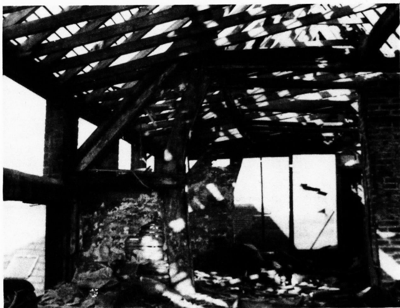
Old and new roof structures at 17—19 London Street. The steep pitch of the original roof is apparent, its structure hidden behind a modern roof supported by brick pillars. (J.K. Major).
