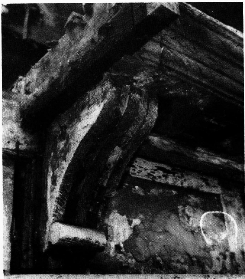
Elegance in decay: A detail of one of the brackets which supported the jetty. (J.K. Major).
